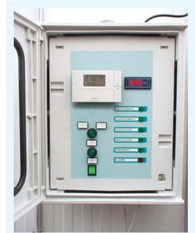
Temperature and humidity control in the whole room for homogeneous germination.
